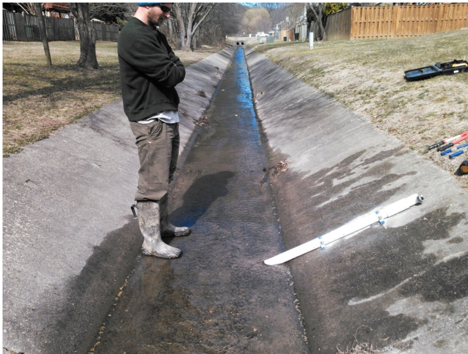
Figure 18. Installation of pressure transducers at monitoring location SC.
